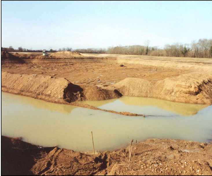
Plate 1: Dewatering excavations at Stonecastle Farm Quarry
